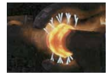
Conventional way of gas pressure welding joints
